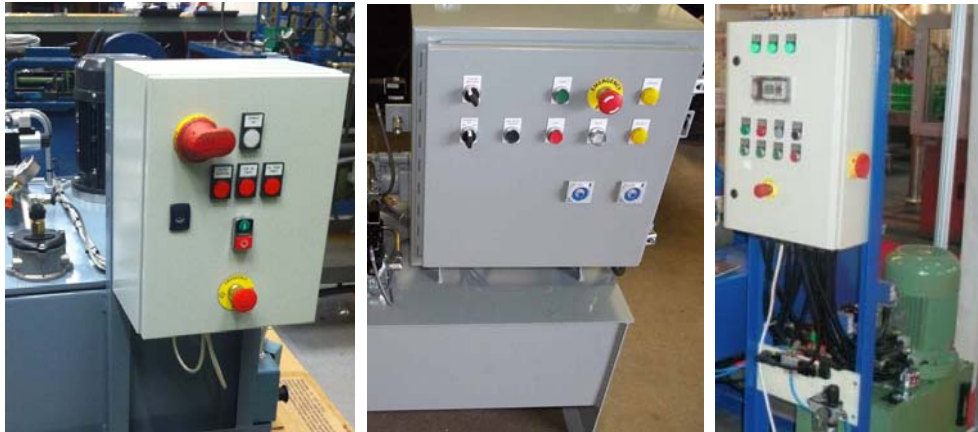
Figure 1. Typical examples of hydraulic aggregates' control units
