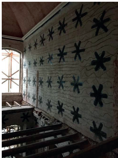
Figure 18-19. Strengthening of brick wall and dome with carbon fiber material.
