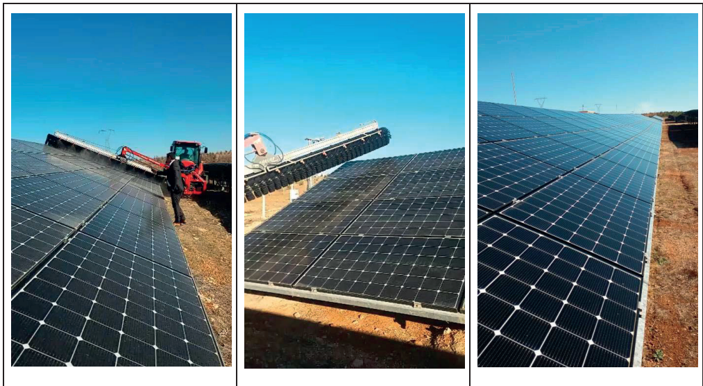
Figure 2. Washing dirty panels with a wet washing machine from the field
