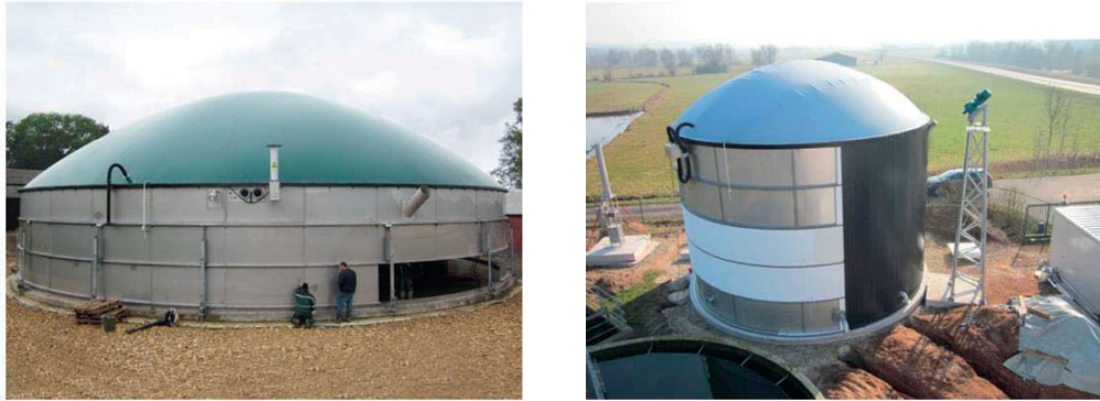
Figure 9. Stainless steel fermenter under construction.
