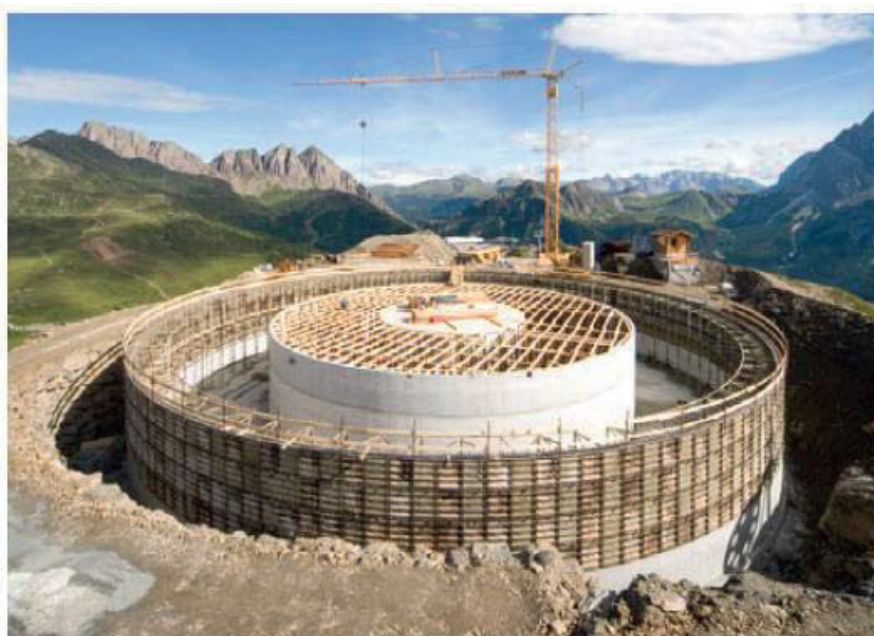
Figure 8. Construction of a concrete fermenter
