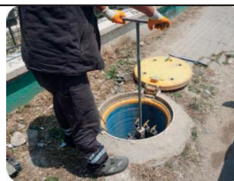
Figure 5. Embedded Valve Control
