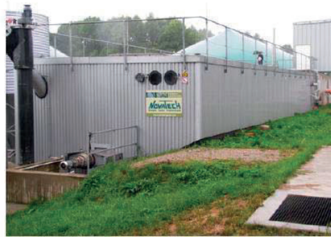
Figure 7. Fermentor with reciprocating flow; examples from practice, cylindrical (left) and rectangular (right).
