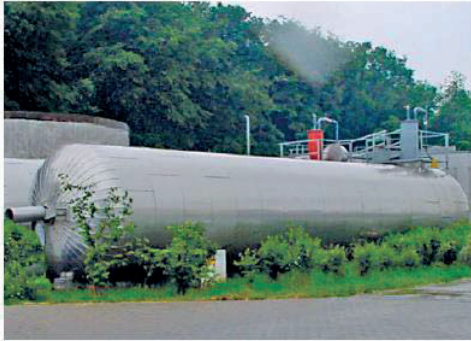
Figure 7. Fermentor with reciprocating flow; examples from practice, cylindrical (left) and rectangular (right).
