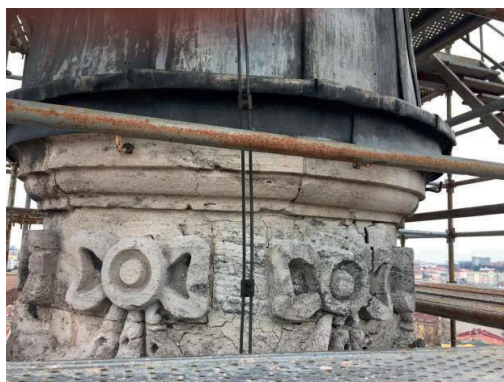
Figure 8. Deterioration of lead covering and stone. Figure 9. Restored lead covering.
