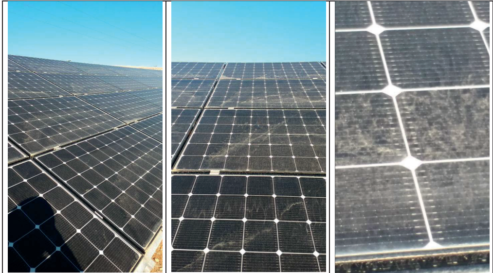
Figure 1. Dirty PV panel images from the field
