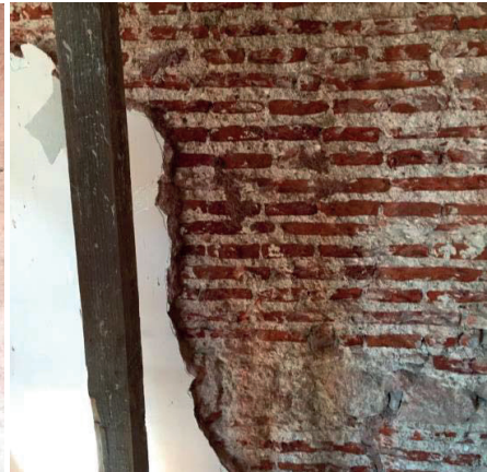
Figure 11. Brick deterioration.
