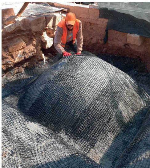
Figure 18-19. Strengthening of brick wall and dome with carbon fiber material.
