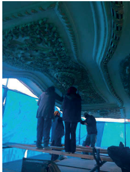
Figure 14-15. Consolidation of decorations with simple repair and strengthening.
